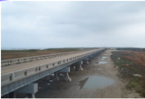
Figure 3 The San Luis Pass low-level bridge that is subject to tidal conditions, high in chloride ions.
